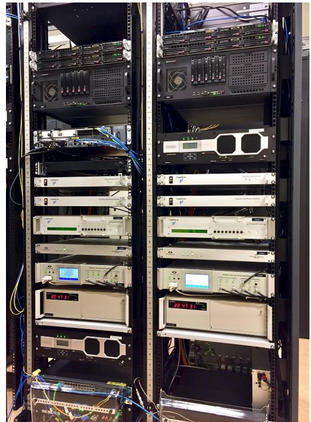
Fig. 3. A time node, with cesium clocks (red displays), phase and frequency steppers (blue-white displays), distribution amplifiers, multi-channel time interval counters for monitoring, GNSS receiver, PTP grandmasters, and computers. The taller computers close to the top are the NTP servers.
