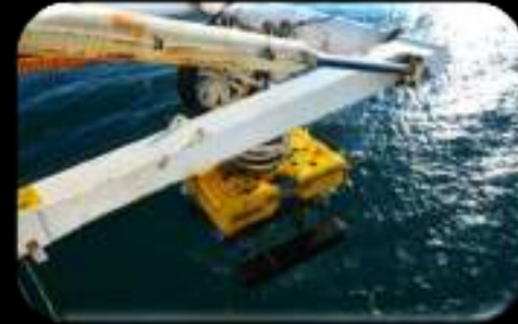
ROV control after cable lay
